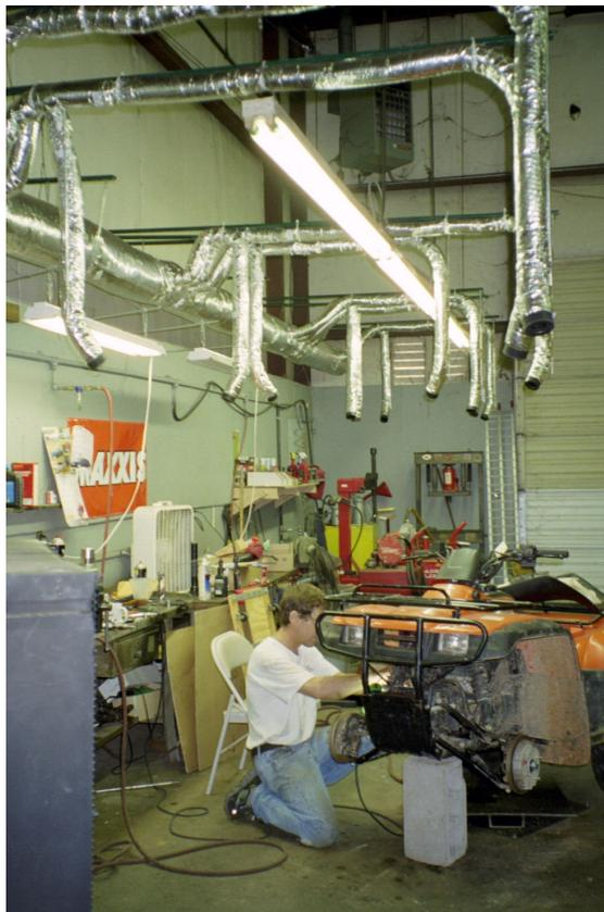
*3 or 4 spot cooling outlets extend down to each workstation allowing the service mechanic to stay cool as he works.*
