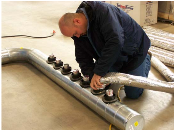
Niel Gerrald of Aloha Air in Texarkana, Texas, connects the supply tube to the plenum during a Unico training session sponsored by R.E. Michel.
