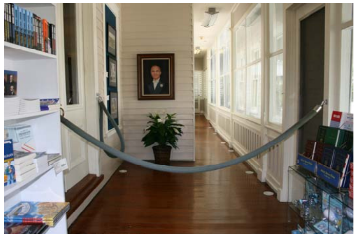
Circular Unico outlets were installed in the wood floor.
