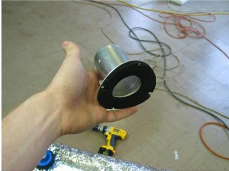
**STEP 2.** Attach Take-off directly to insulated plenum using four sheet metal screws
