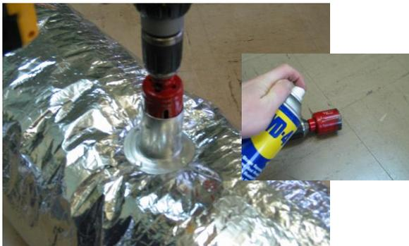
**STEP 4.** Visually inspect the hole for any excess metal or insulation.
