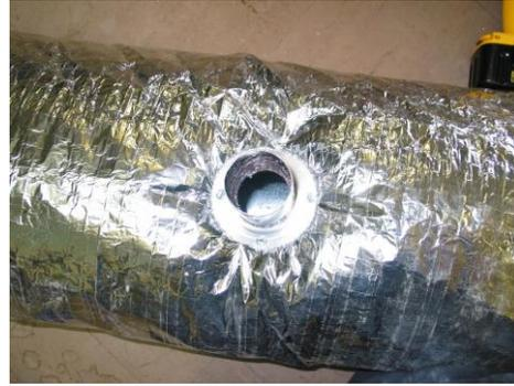
**STEP 5.** Peel the adhesive backing from the underside of the overlay gasket, slip it over the take-off and stick it to the vapor barrier. Apply even pressure around to secure.
