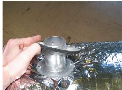
**STEP 6.** Once the gasket is sealed against the insulation vapor barrier, peel off the backing on the top side to secure the tapering in the next step.
