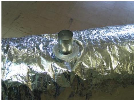
**STEP 3.** Use a 1-7/8-inch diameter hole saw (with extension if necessary) to cut through the insulation and duct.
