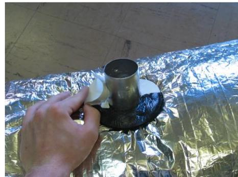
**STEP 7.** Slip the tape ring over the take-off and seal it against the gasket, then connect the branch duct using a clamp and seal the outer vapor seal against the tapering with UL tape.
