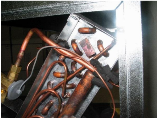
Figure 26. (Step 5) Route both the pressure and temperature tubes as shown.
