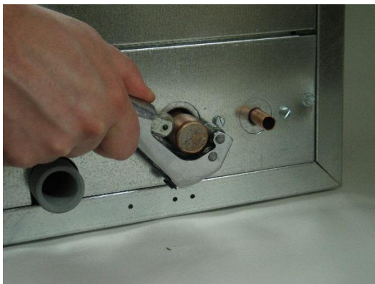
Figure 21. Cut end of connection as shown.
