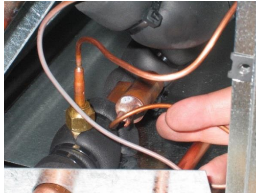
Figure 28. (Step 7) The thermal measuring bulb is placed as shown. It needs to be in contact with copper tube.
