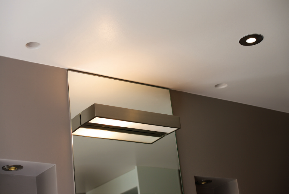
All supply outlets were plastered into the ceilings, leaving just discreet 2-inch holes delivering the conditioned supply air. This sleek look could not have been achieved with a traditional heating and air conditioning system.
