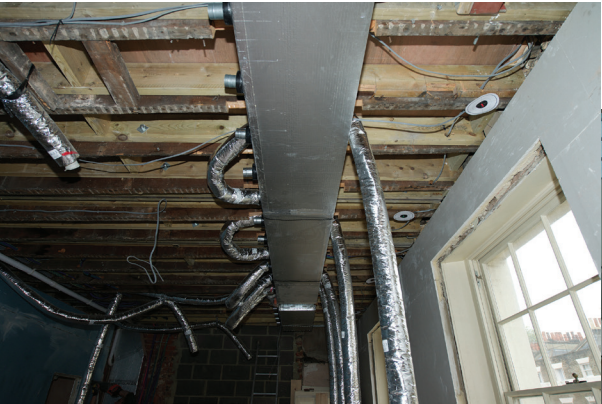
The Unico System main trunk line and supply ducts. Note: the templates used to ensure proper location of the terminating outlets.
