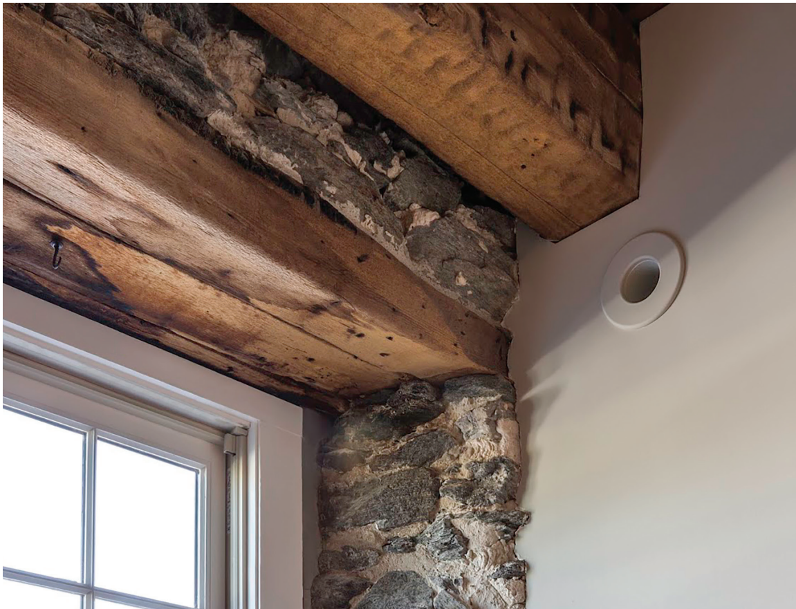
A.P. Whitaker & Sons' project manager, Paul Lacey, put a lot of time and effort into finding wood that would match the original post-and-beam exposed woodwork.
