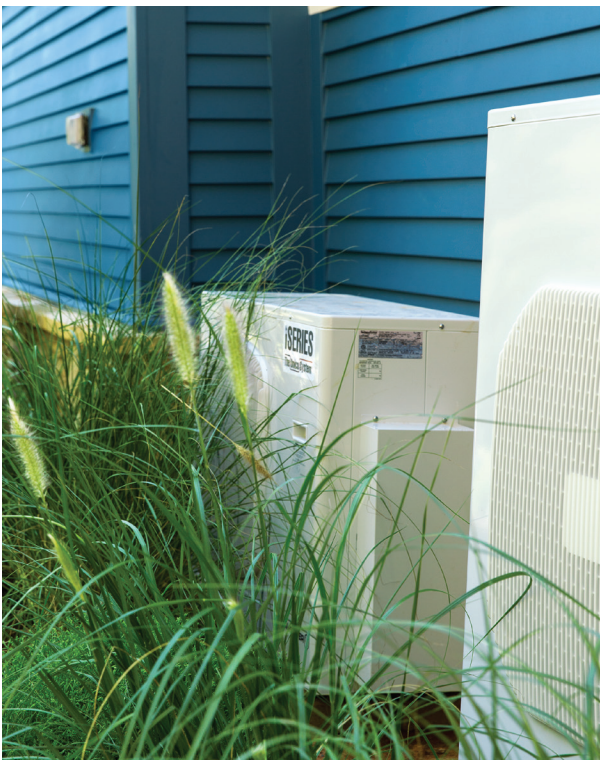
The Unico iSeries heat pump features inverter technology for highly efficient heating and cooling.
