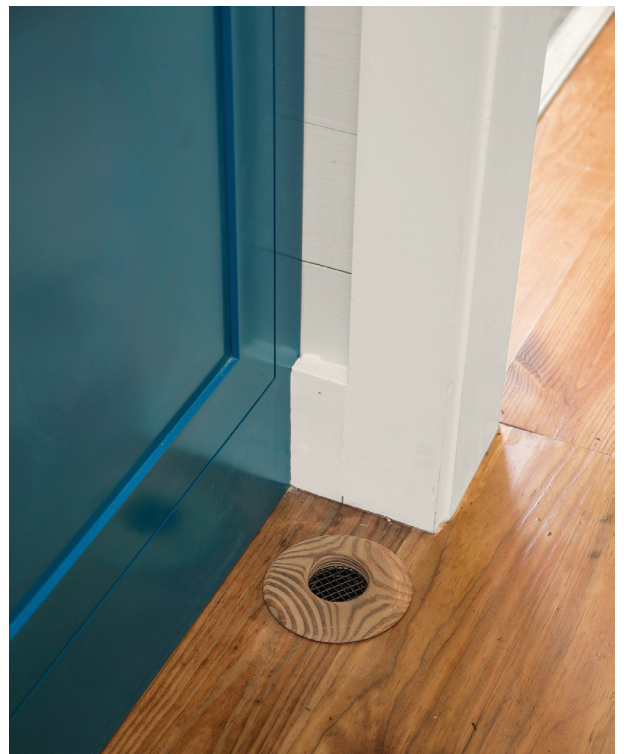
Unico room outlets can be stained or painted to match any décor.
