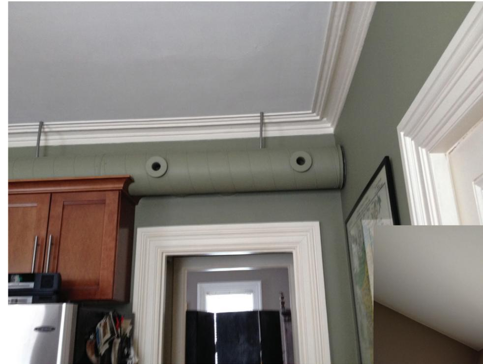
Supply tubes are routed through spiral duct for an industrial look in the kitchens of the 1st and 2nd floor apartments.
