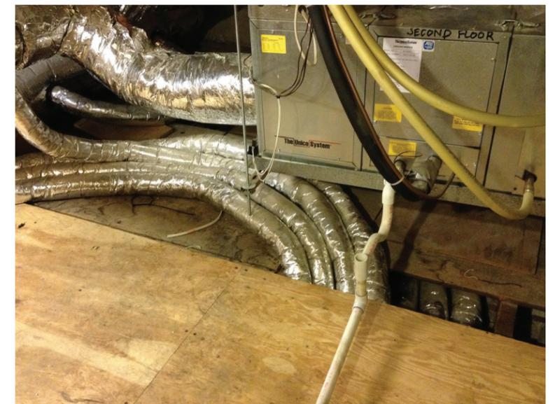
Air handling equipment and main trunk lines for the 2nd and 3rd floor apartments are housed in the attic.
