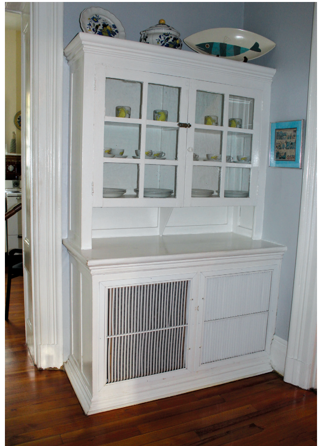
This retrofitted cabinet hides the return air box.
