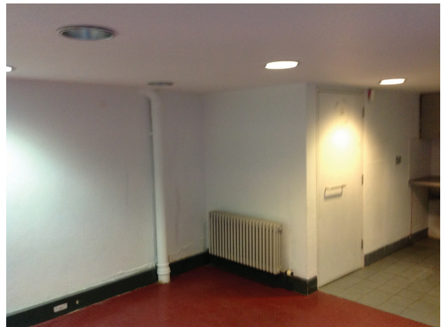
Before the renovation, radiators provided heat to the lower level, while a high-wall mini-split provided cooling.
