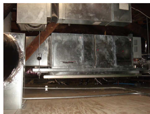
Unico blower and coils in attic
