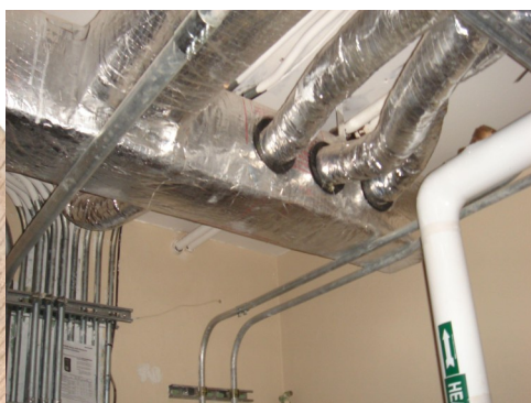
Supply ducts coming off main plenum
