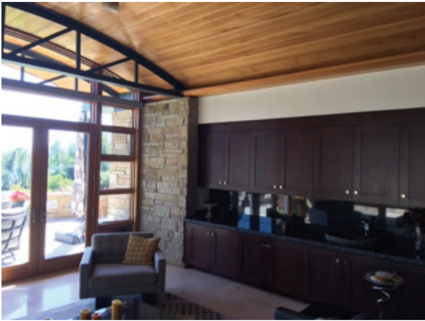
The barrel vault ceilings of this custom home would not allow for the inclusion of conventional HVAC without major alterations for ductwork concealments.
