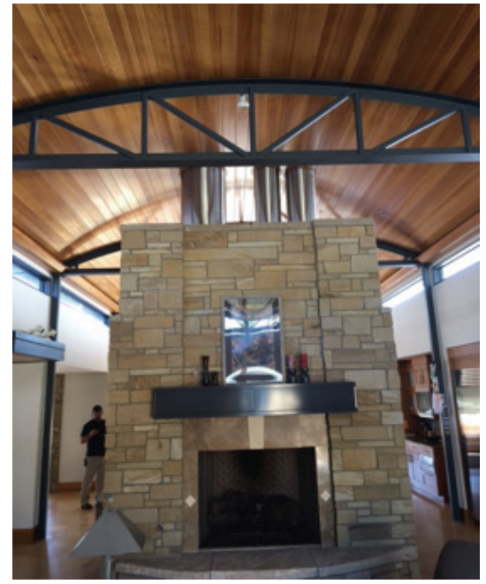
Unico supply tubing is concealed within the stainless-steel exhaust ducts embedded in the open, flagstone fireplace.
