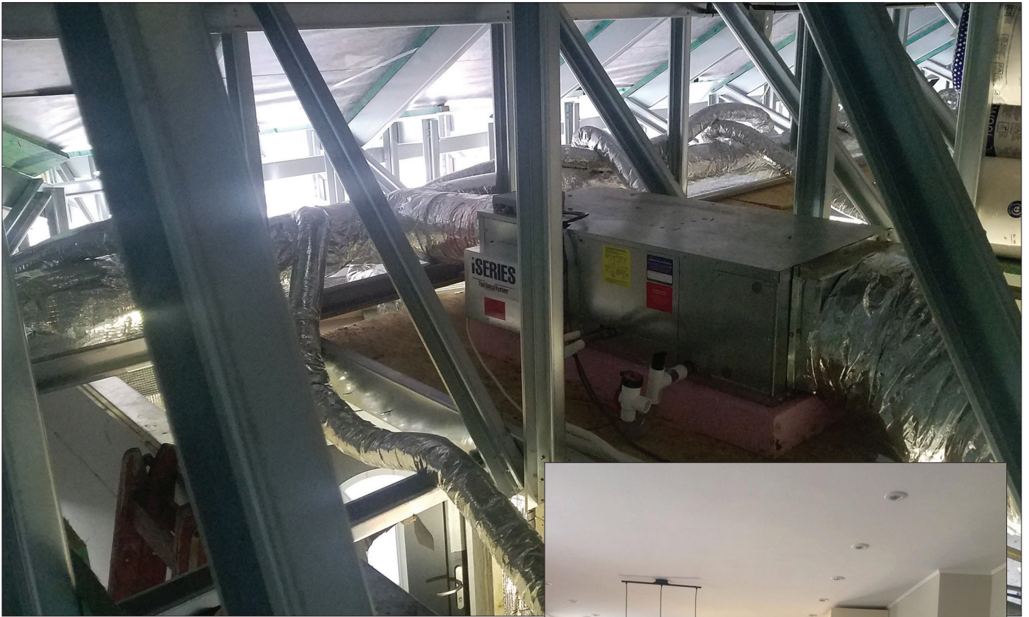
The air handling unit and main trunk ducting are located in the attic and feed the round ceiling outlets with flexible supply tubing.
