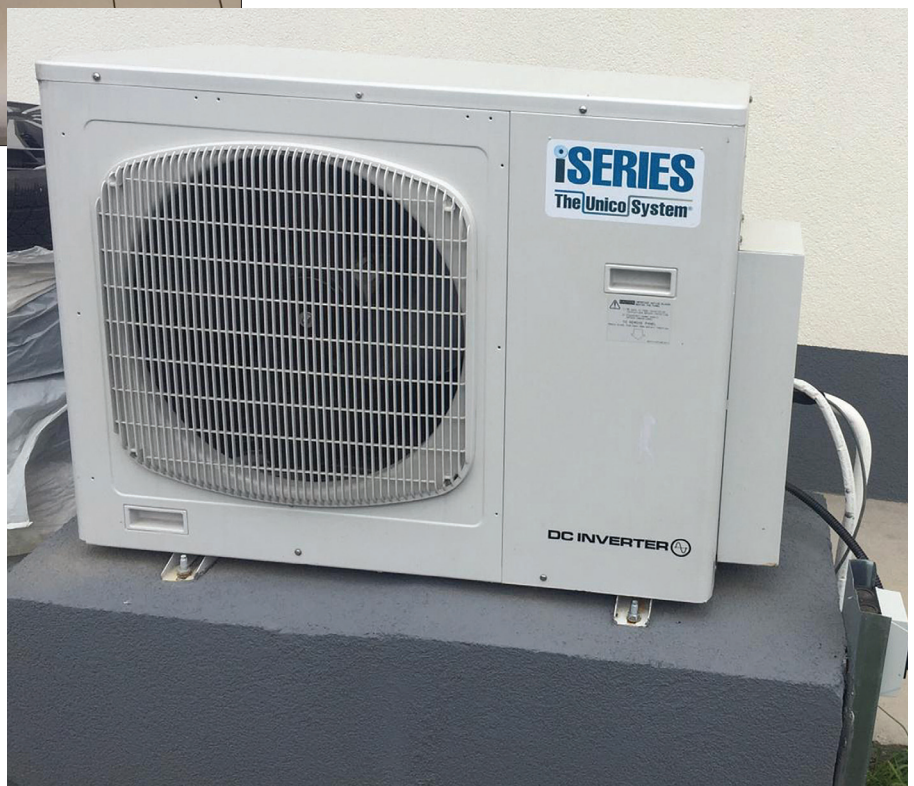
The Unico System iSeries inverter heat pump is the outdoor component of the HVAC system. Electric inverters are highly efficient means of supply heating and cooling.
