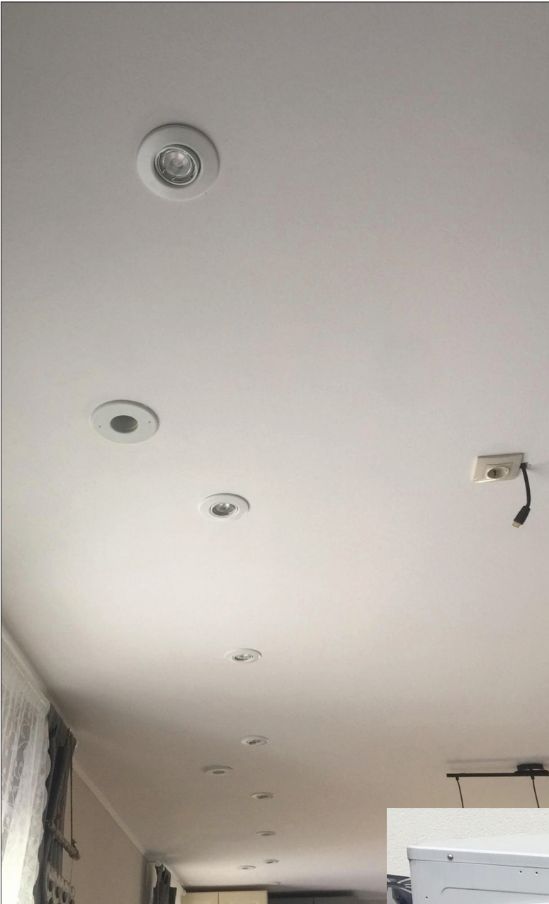
Unico System round outlets terminate in the ceiling and blend in with the lighting fixtures.
