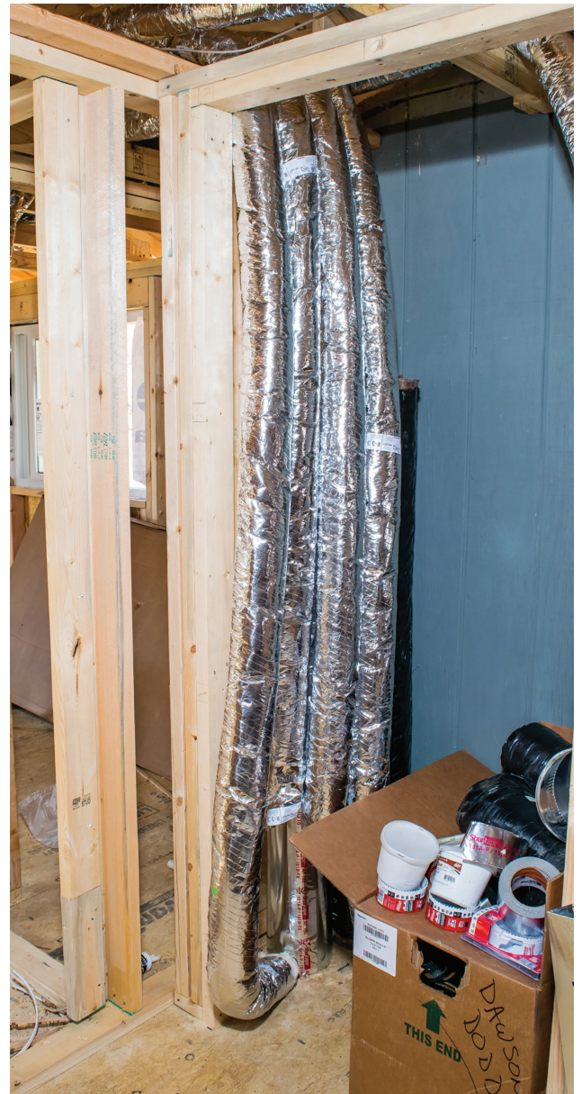
Four flex ducts being built into a closet wall (leading from the attic to the main floor).
