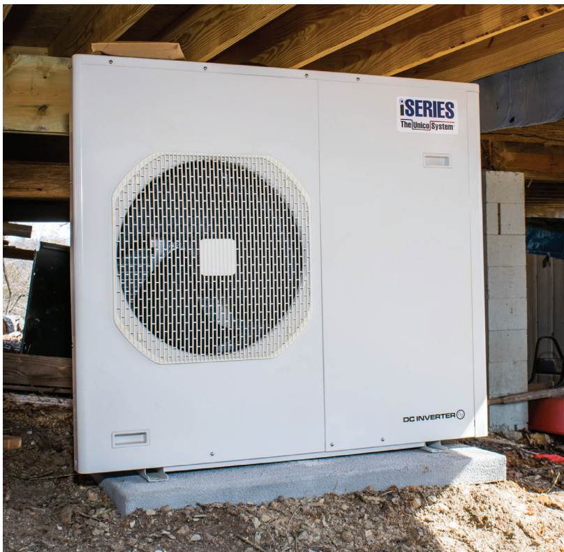
Unico i-Series (3-ton unit), installed near the master bedroom.
