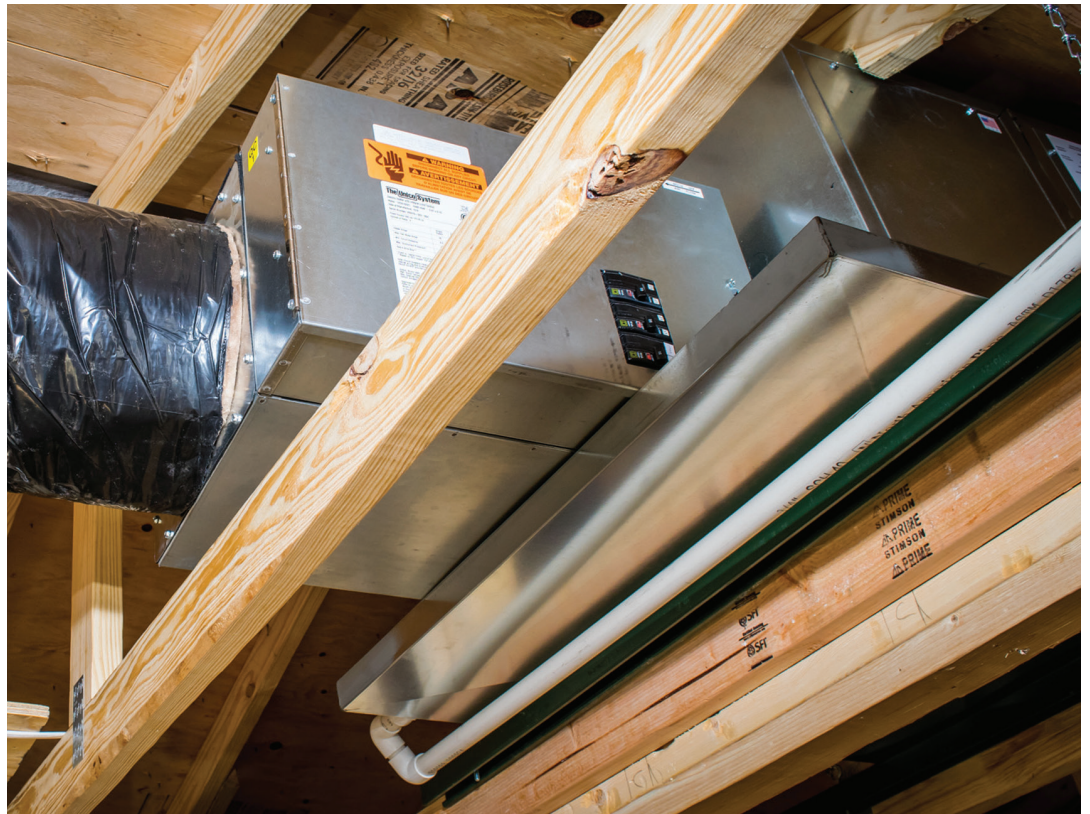
Main trunk line with flex ducts above the ceiling of the top floor.
