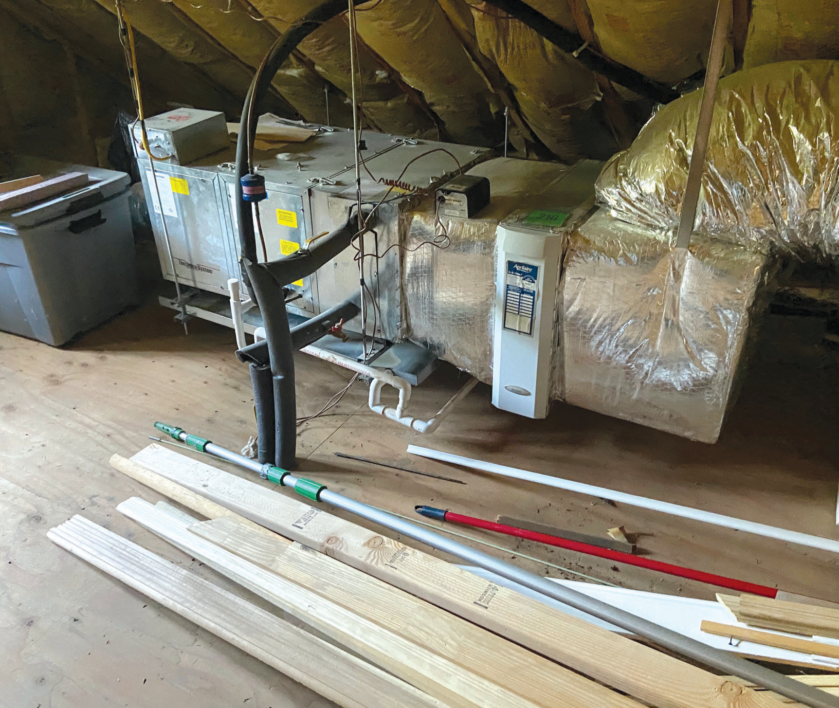
The Unico System air handling equipment and main trunk located in the attic.
