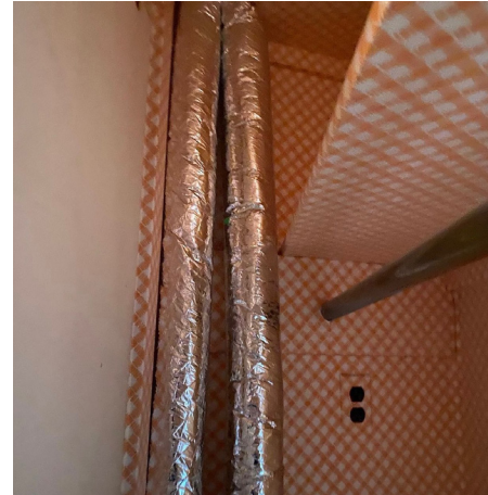
Flexible supply tubing was also routed through the negative space of some closets.
