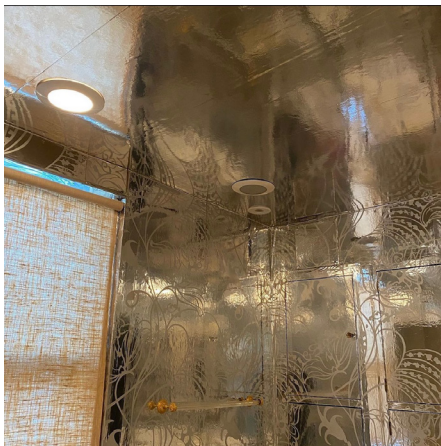
Outlets were installed with care so as not to damage the unique but brittle foil wallpaper in the master bedroom.
