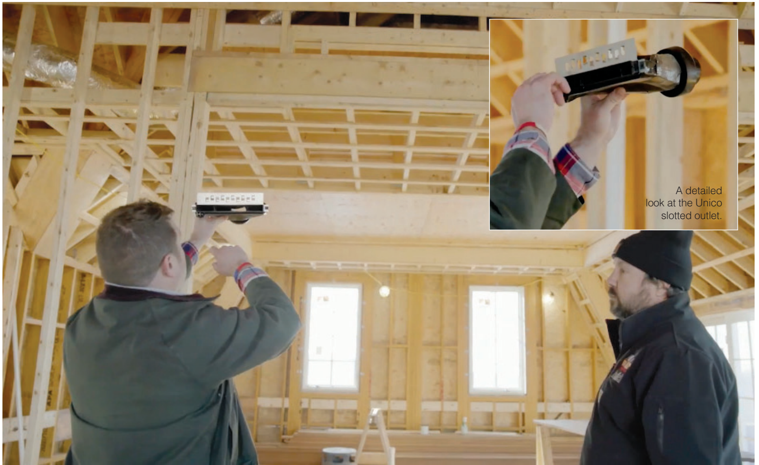
Evan demonstrates to Wade how Unico slotted outlets will be placed side-to-side, along the tray ceiling then finished to virtually disappear as one long ½-inch high slot opening.
