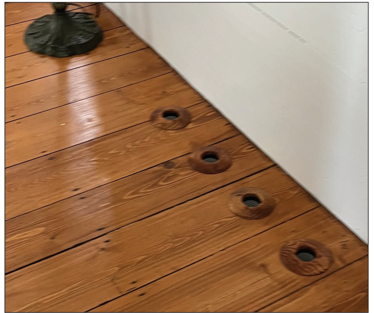
Unico's discreet round outlets were stained to match the color of the original plan flooring.
