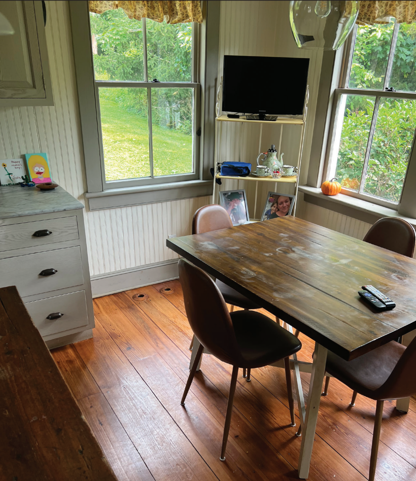
Unico's discreet round outlets were stained to match the color of the original plan flooring.
