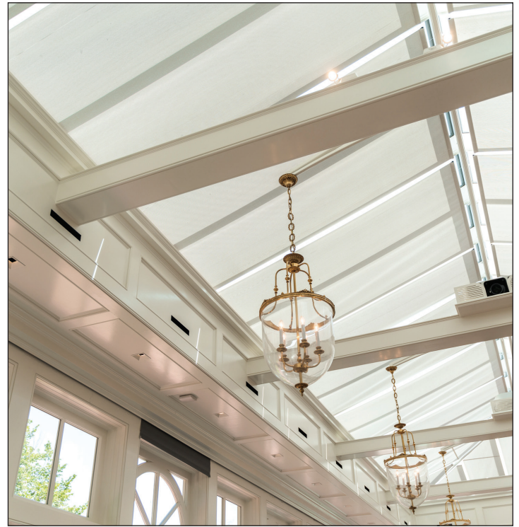
These custom-designed rectangular openings provide whisper quiet heating and cooling for this nearly all glass addition.
