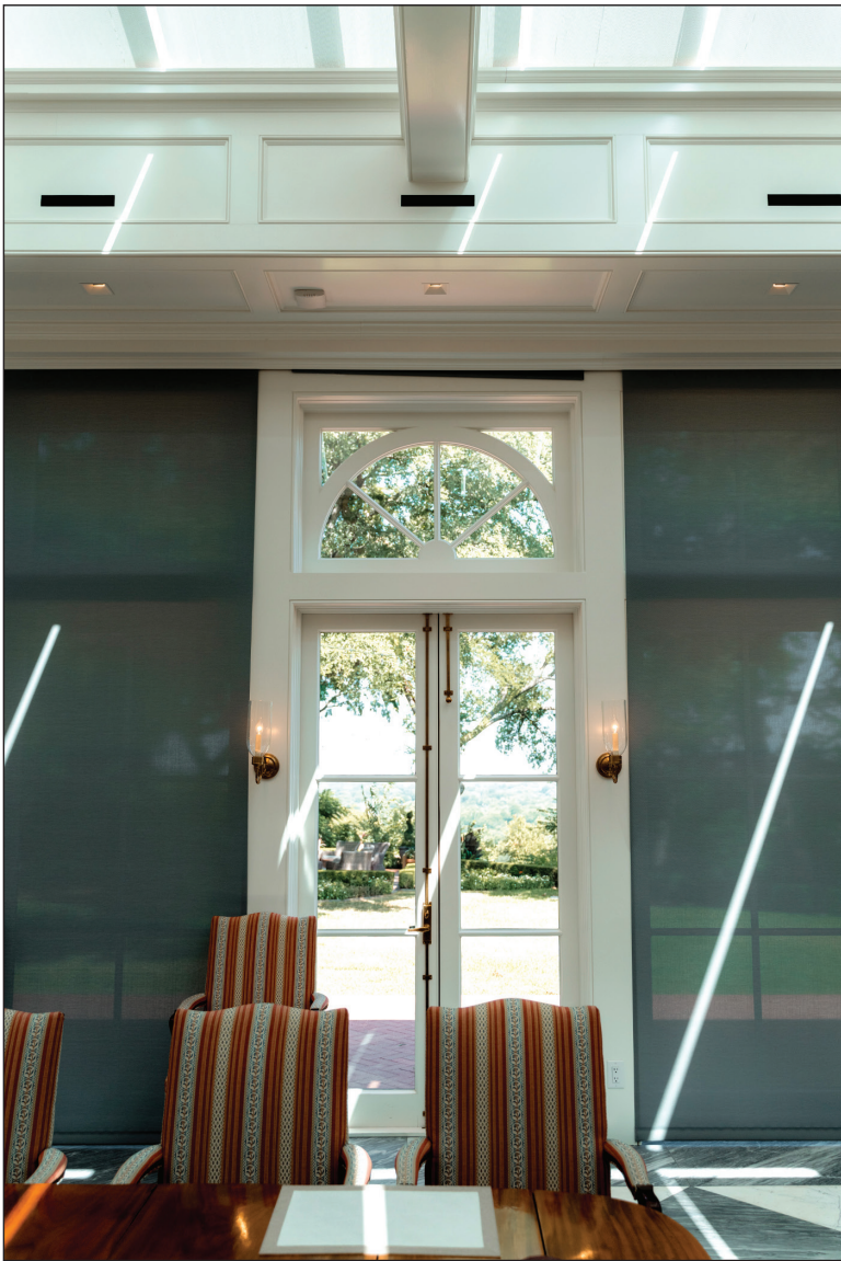
These custom-designed rectangular openings provide whisper quiet heating and cooling for this nearly all glass addition.
