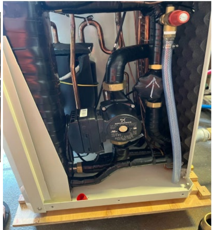
Removing the shipping spacer
