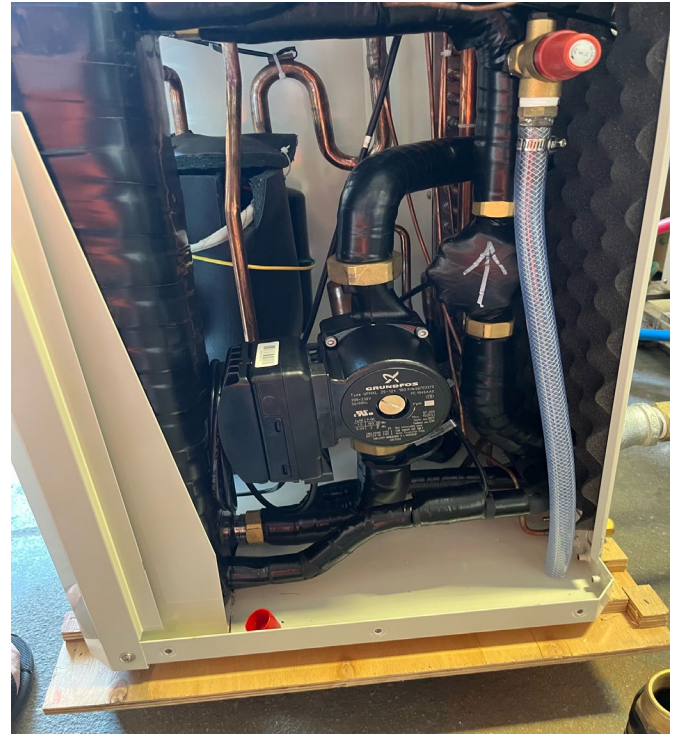
Removing the shipping spacer
