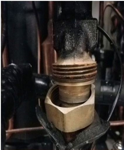
Peel back the insulation
