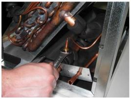
Figure 28. Tighten Pressure Tube Nut
