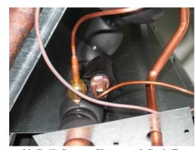
Figure 30. Bulb Secure Clamp and Cork Tape
