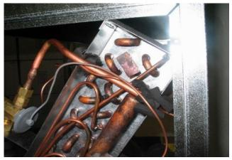
Figure 27. External equalizer line and themostatic bulb line location routing
