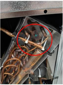
Figure 24. Cut zip ties before installing TXV
