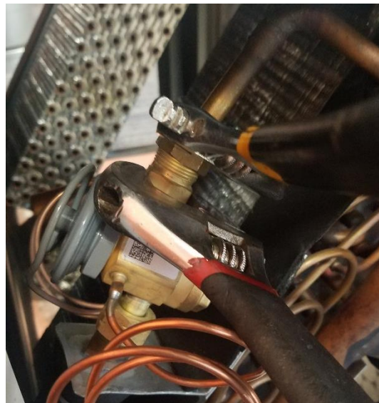
Figure 10. Attaching TXV to Liquid Line
