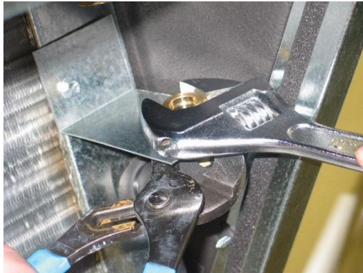
Figure 23. Remove Nut
