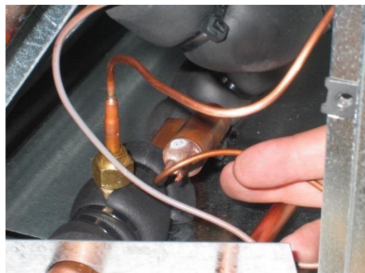
Figure 29. Thermal Measuring Bulb Placed on Copper Tube.
