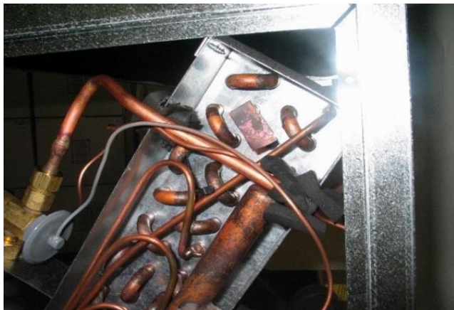
Figure 27. External equalizer line and thermostatic bulb line location routing
