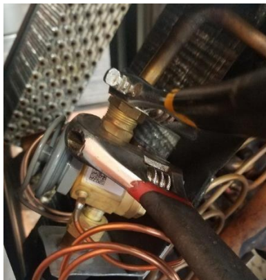
Figure 26. Attach and tighten upper connecting nut (B/E coils)
