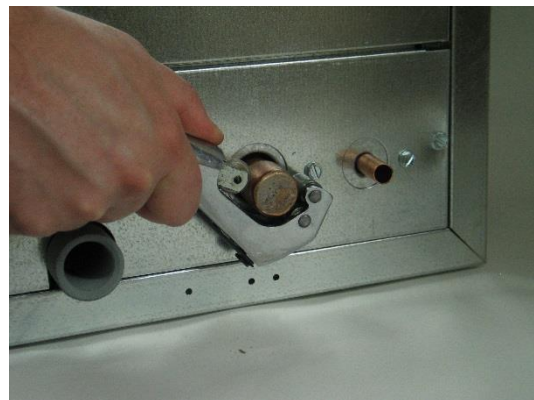
Figure 22. Cut end of connection as shown.
