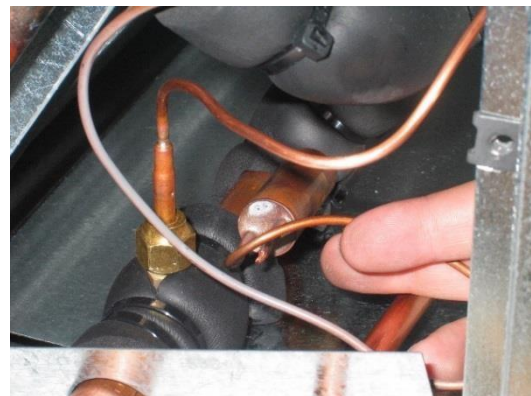
Figure 29. Thermal Measuring Bulb Placed on Copper Tube.
