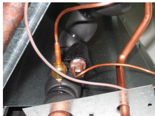
Figure 30. Bulb Secure Clamp and Cork Tape
