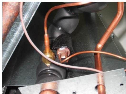
Figure 30. Bulb Secure Clamp and Cork Tape
