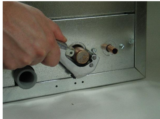
Figure 22. Cut end of connection as shown.
