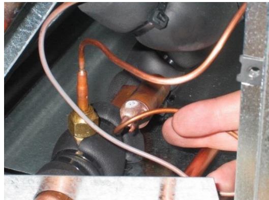
Figure 29. Thermal Measuring Bulb Placed on Copper Tube.
