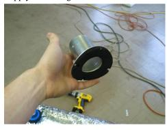
**STEP 2.** Attach Take-off directly to insulated plenum using four sheet metal screws
