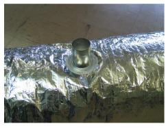
**STEP 3.** Use a 1-7/8-inch diameter hole saw (with extension if necessary) to cut through the insulation and duct.
