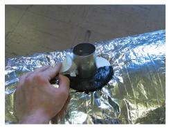
**STEP 7.**Slip the tape ring over the take-off and seal it against the gasket, then connect the branch duct using a clamp and seal the outer vapor seal against the tapering with UL tape.
