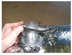
**STEP 6.** Once the gasket is sealed against the insulation vapor barrier, peal off the backing on the top side to secure the tapering in the next step.
