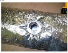
**STEP 5.**Peal the adhesive backing from the underside of the overlay gasket, slip it over the take-off and stick it to the vapor barrier. Apply even pressure around to secure.
